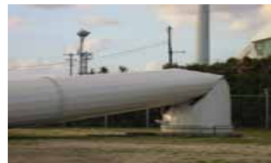
Collapsed due to the buckling of the tower
