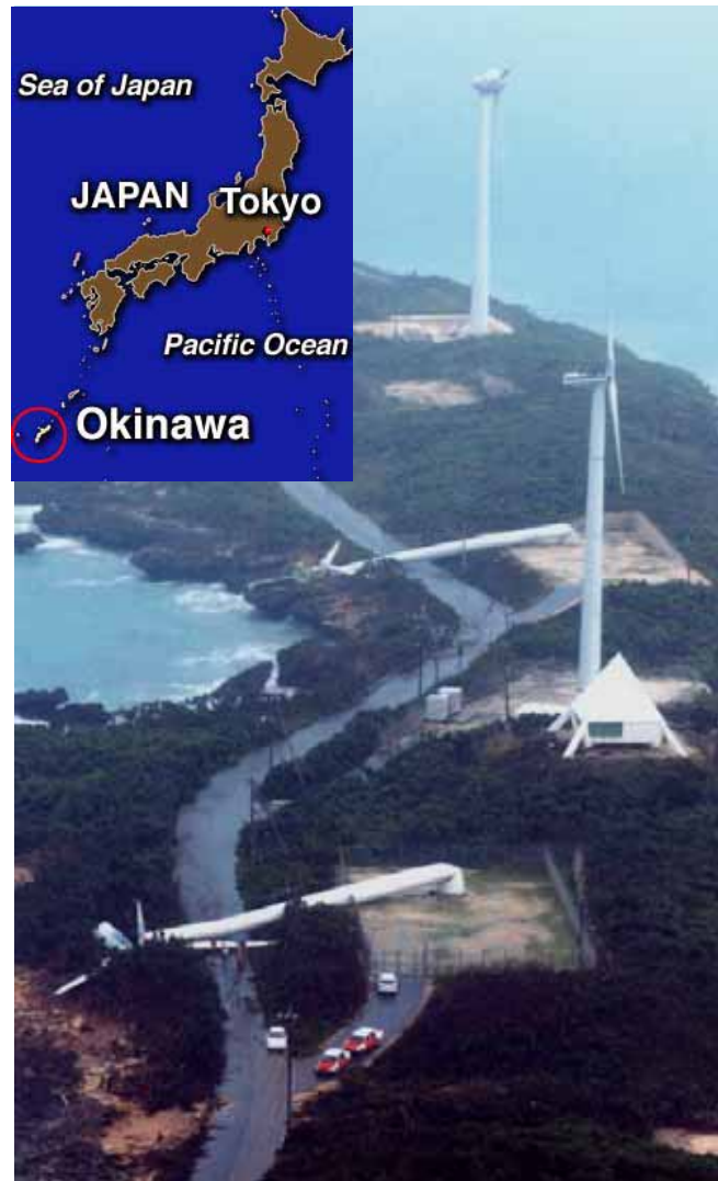
The damage of turbines in the Okinawa Island by typhoon Maemi in 2003
