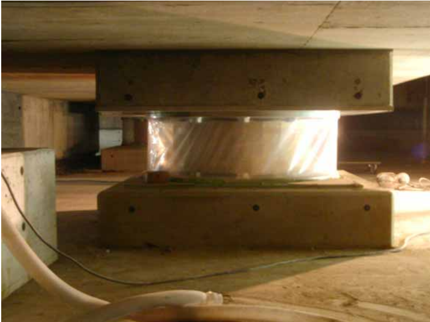
Device of Base-Isolation Scheme (Rubber Bearing)
